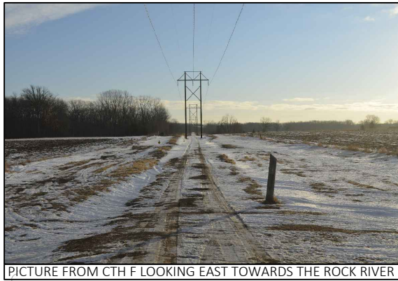
PICTURE FROM CTH F LOOKING EAST TOWARDS THE ROCK RIVER
